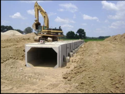
Box Culvert Construction
