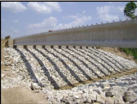
Concrete Beams for Bridge 3
