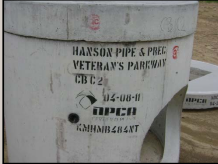
Drainage Structures on Site
