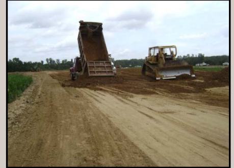
Earthwork near Bridge 2
