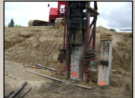
Pile Driving at Bridge 3
