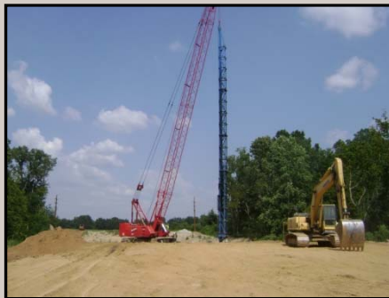
Pile Driving at Bridge 1
