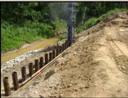
Pile Driving at Bridge 1
