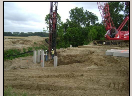
Pile Driving at Bridge 3
